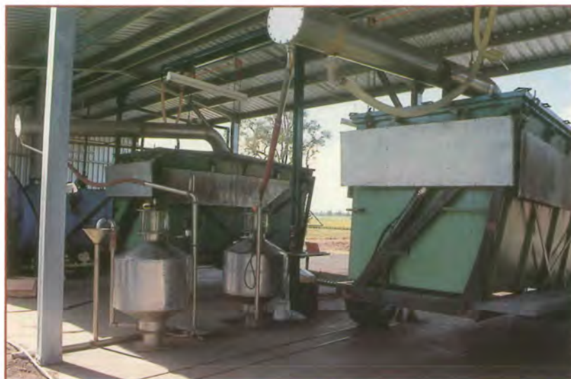
Tea tree oil processing plant at Coraki
