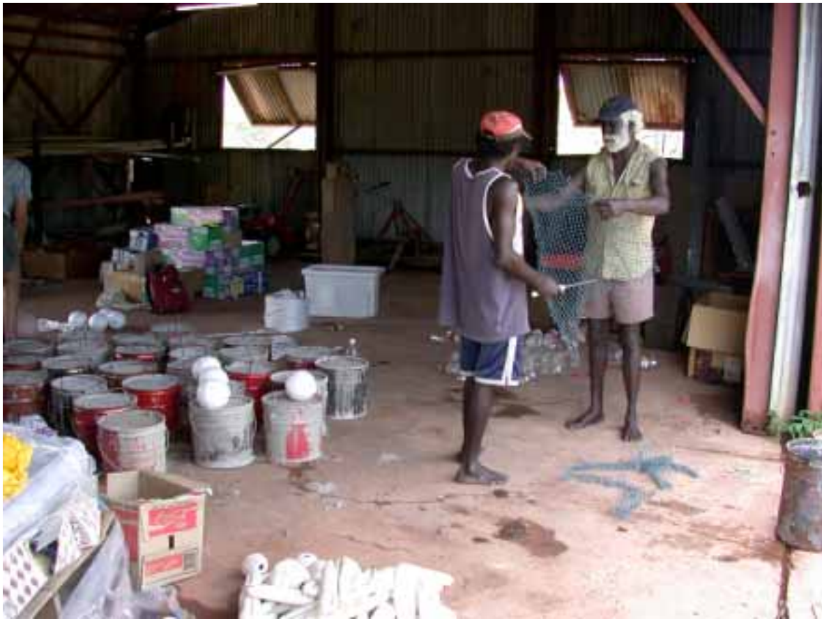
Figure 2. Roy and Henry of the Warruwi Sea Rangers recycling old material to use in the sponge farming experiment. Also shown are the 20 kg anchor weights, made from flour containers filled with concrete.
