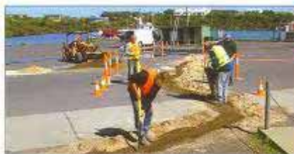
Workmen installing the surveillance equipment at the port of Robe, South Australia.
