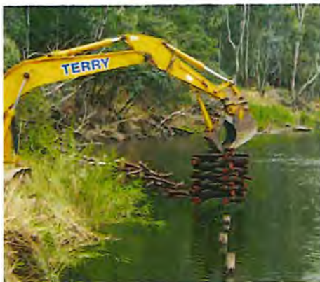
Inserting fish hotels into the Ovens River.
