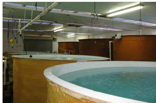
Figure 4 Water storage tanks at Bicheno
