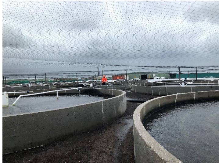
Plate 1. Ten metre diameter culture tanks used during the Jade Tiger Abalone Avalon farm trial.
